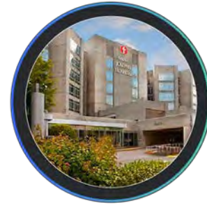
St. Joseph's Hospital Atlanta, GA, USA
